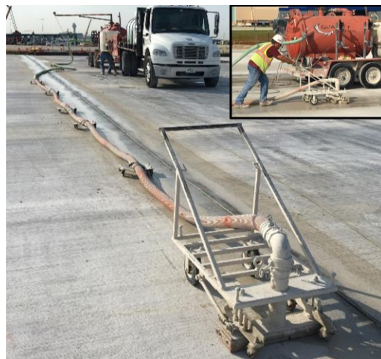
Figure 2 Photo of Wet Saw Vacuum Pickup Equipment
