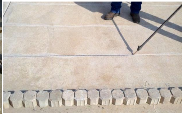
d) Silicone and Hot-pour Seal Placement
