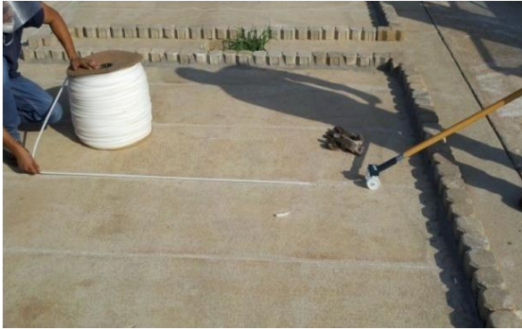
c) Backer Rod Placing
