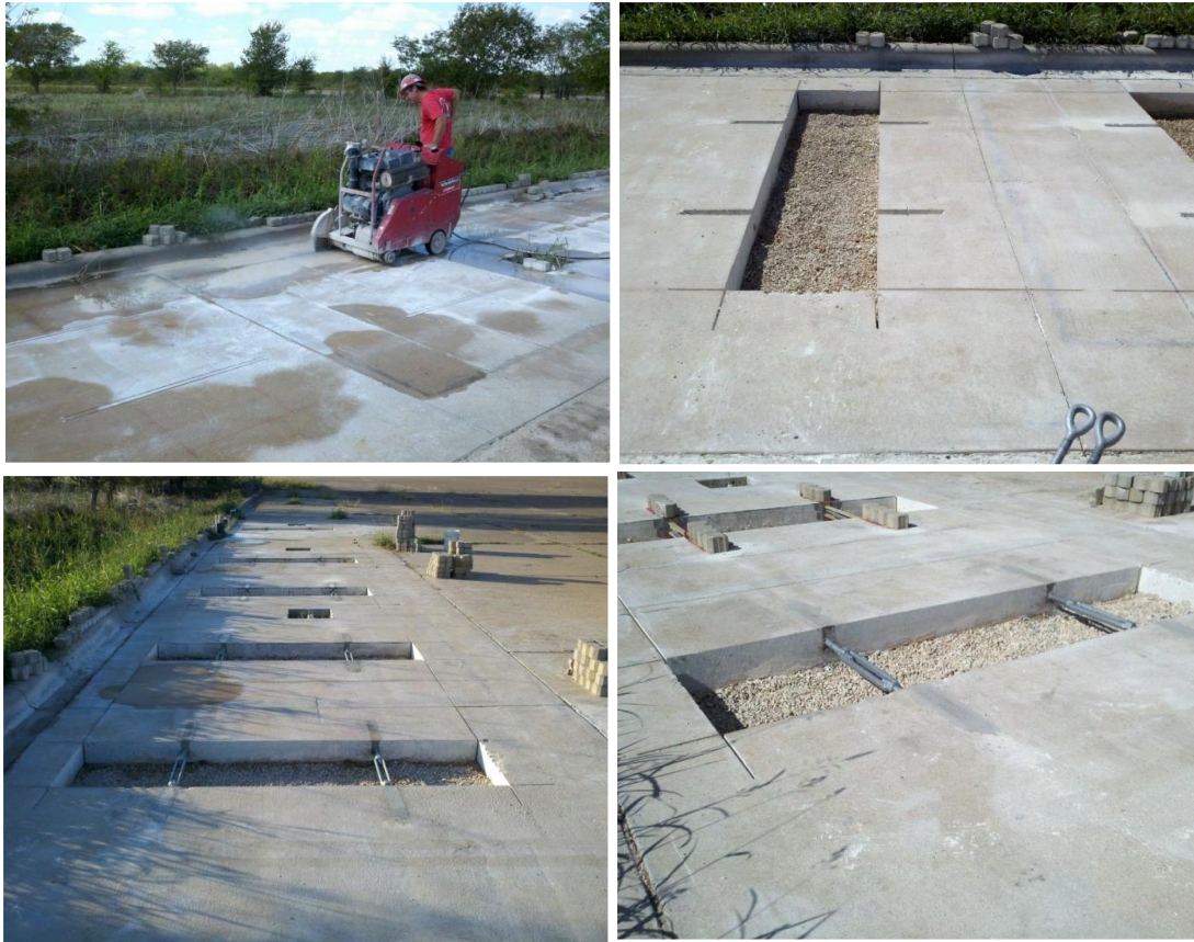
Figure 11 Installation of Movable Joint System.
