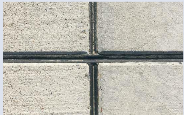
Figure 4 Photo of Properly Installed Compression Seal 2
