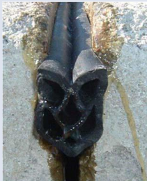
Figure 5 Compression Seal Installed 3
