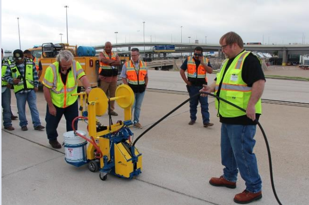
Figure 3 Joint Sealant Installation Equipment
