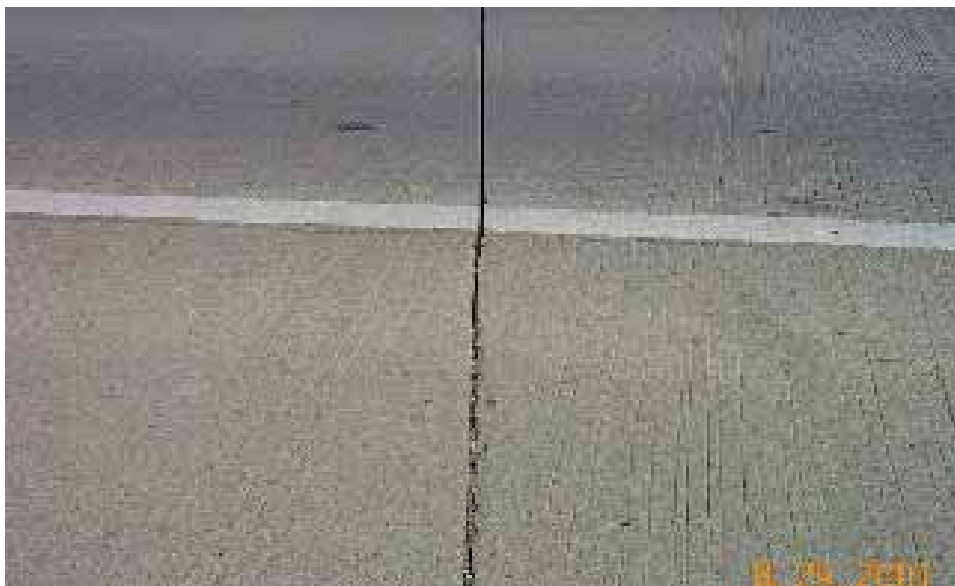
Photo 16 - Incompressible material in shoulder versus driving lane.
