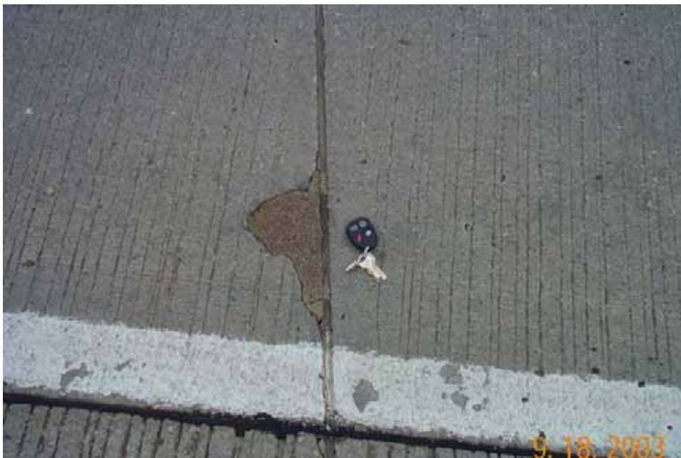
Photo 19 - Attempted spall repair in sealed control section.
