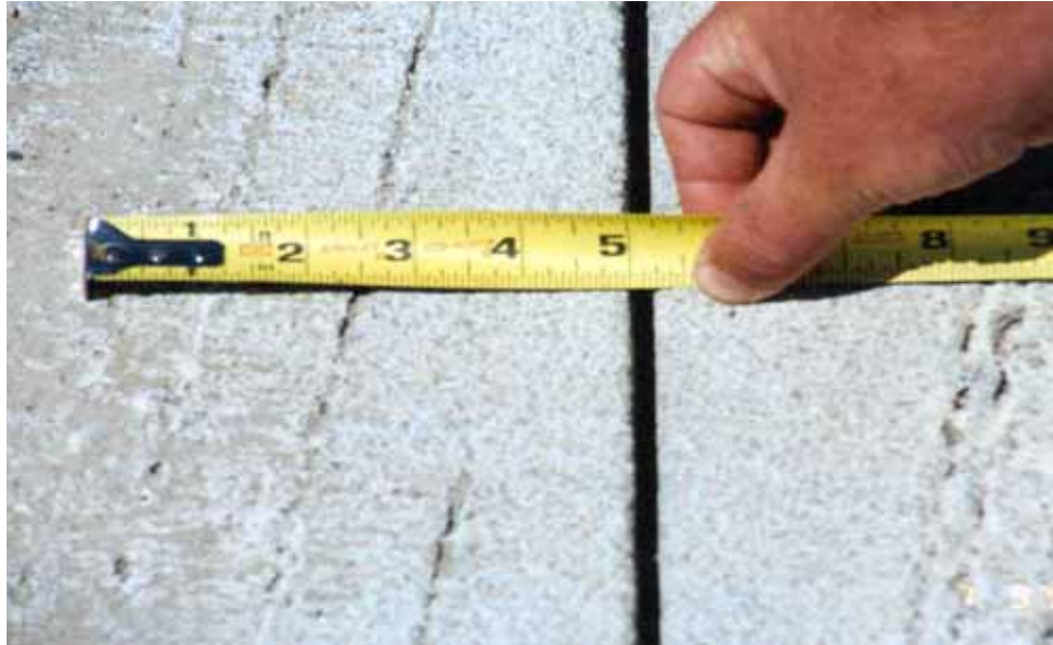
Photo 11 - Close-up view of a portion of an unsealed joint that was sawed correctly.
