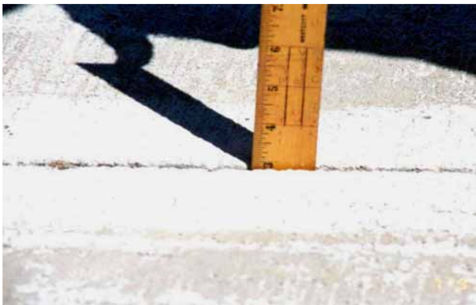
Photo 12 - Saw depth of joint in question to be approximately 3".
