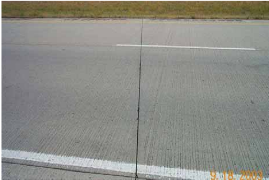
Photo 17 - Typical spalled joint in the test section.
