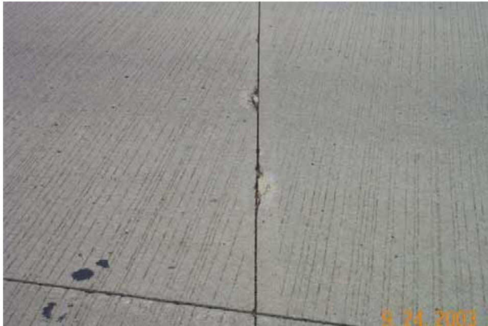
Photo 21 - Attempted spall repair in test section.
