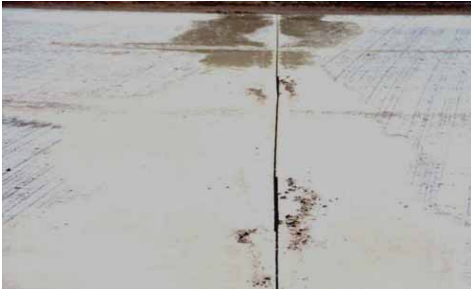
Photo 7 - Extra wide segment caused by the contractors gang saws being out of alignment.
