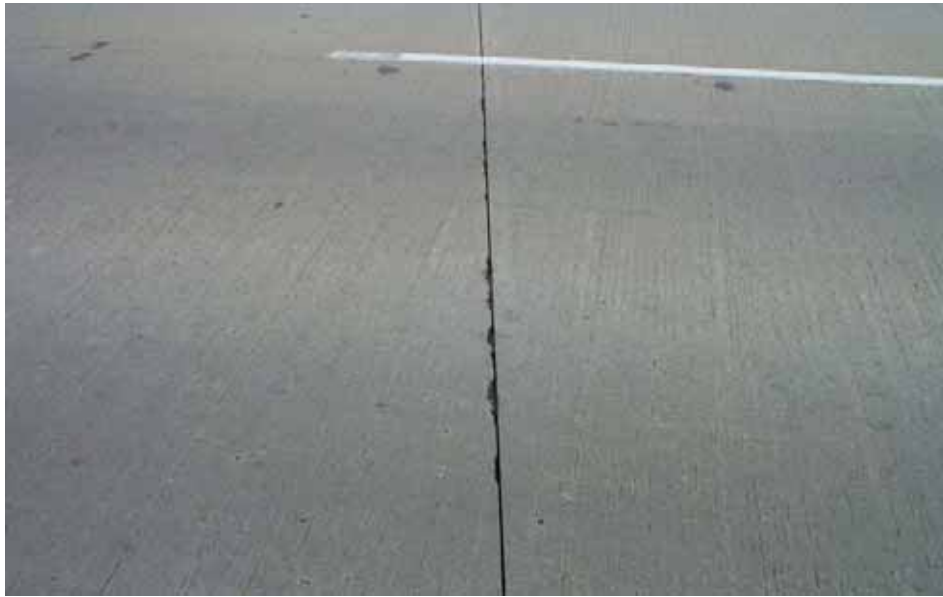
Photo 15 - Most severe spall in unsealed (test) section.
