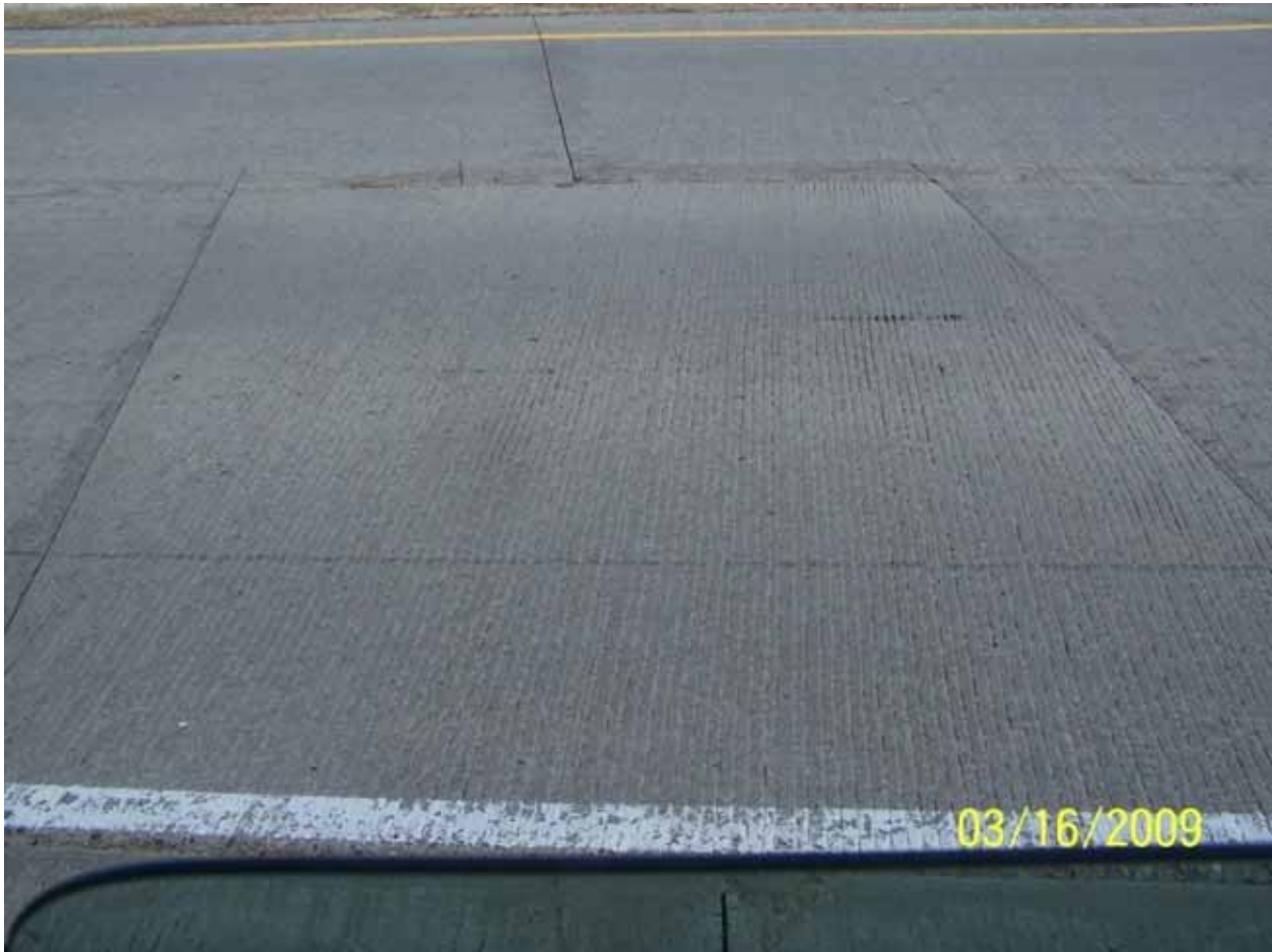
Photo 26 – Photo of repaired joint.
