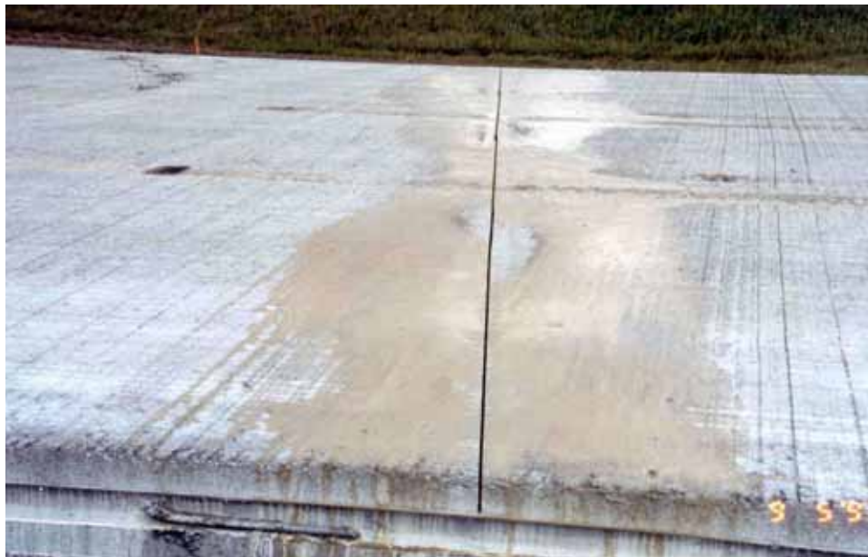
Photo 2 - Typical sawed joint.
