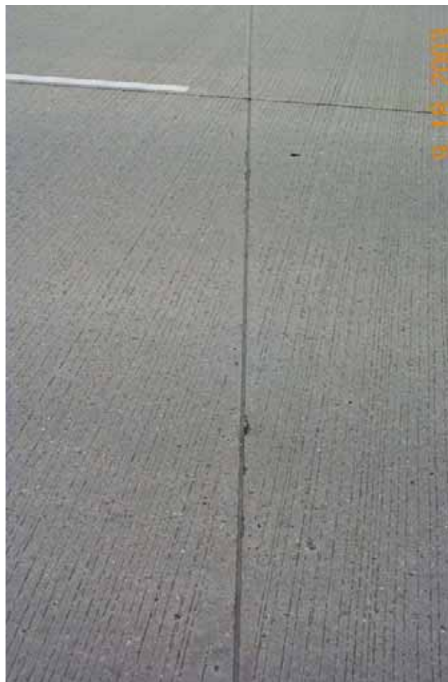
Photo 18 - Typical spalled joint in control section.
