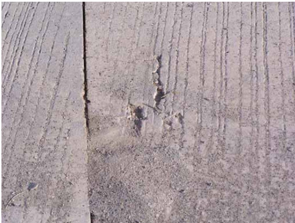
Photo 23 – Photo of severe map cracking next to transverse joint in “control section”.
