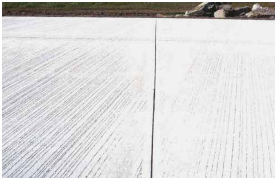
Photo 9 - Typical unsealed joint.
