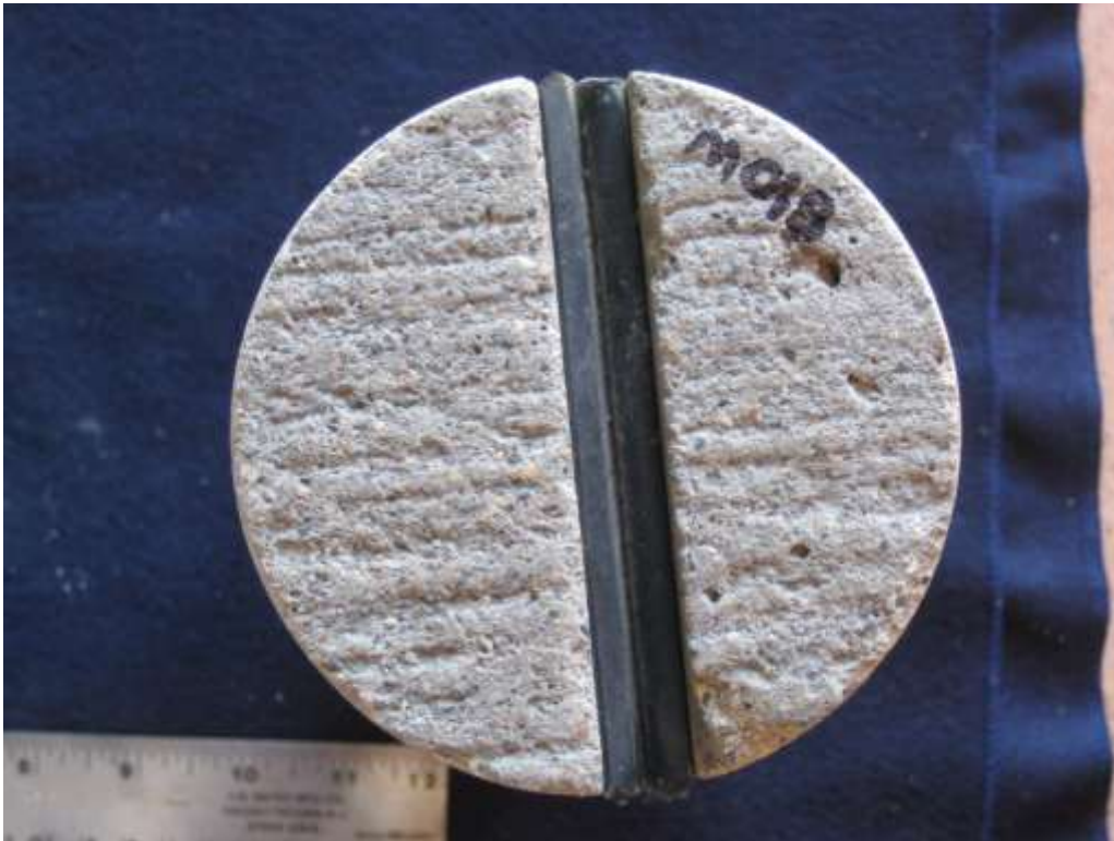
Photo 1: 6" diameter concrete pavement core through a neoprene compression – sealed joint.
