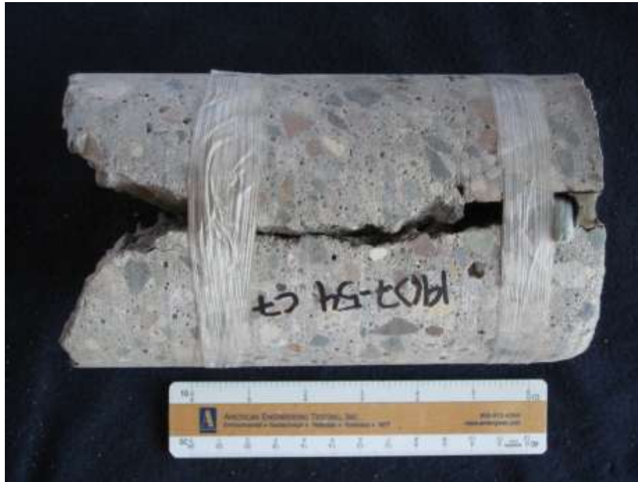
Photo 5: Typical distress pattern in Midwest pavement core through joint. Note conical distress pattern at base of core (L).
