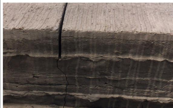
*Development of controlled crack at the transverse joint.*
