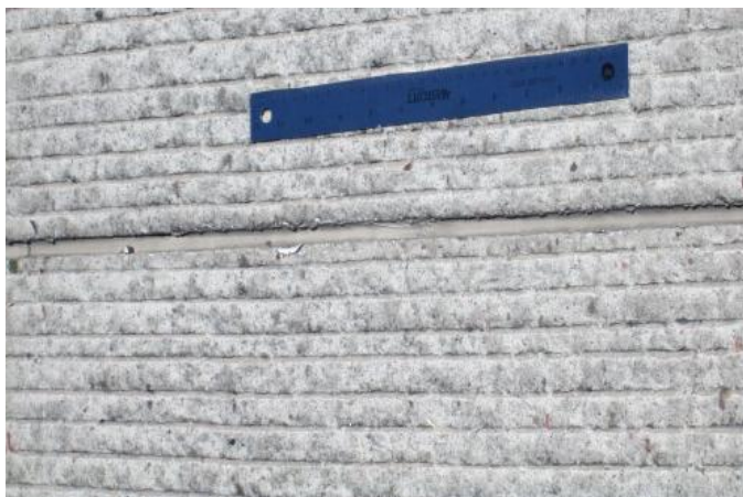
Figure 9. Transverse joint seal in section 222.
