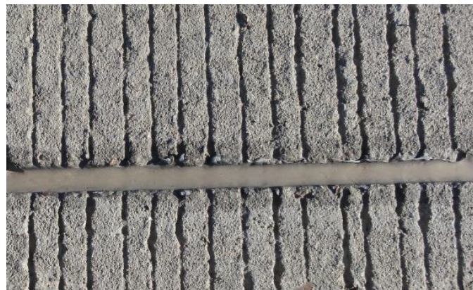
Figure 10. Longitudinal joint seal in section 222.
